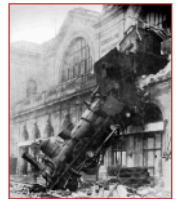
Small errors can lead to big failures.
